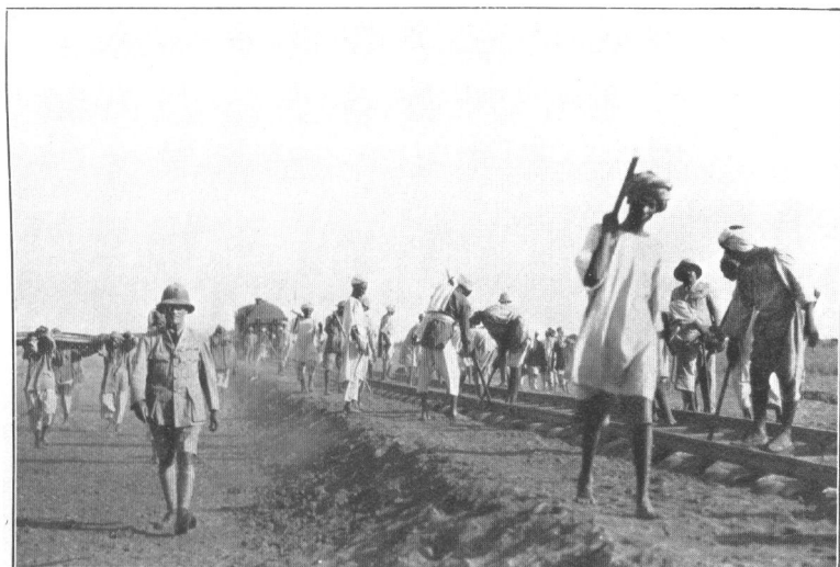
A further stage in the building of the desert railway.
