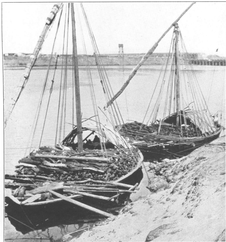
The great Sennar Dam on the Blue Nile in course of construction in April, 1924.
