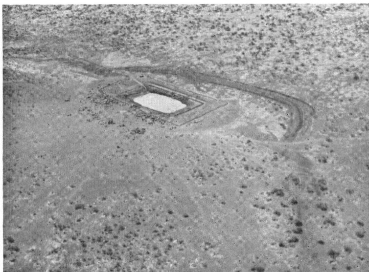
Figure 2. An aerial view of Abu Sana hafir of 25,000 cubic metres capacity
