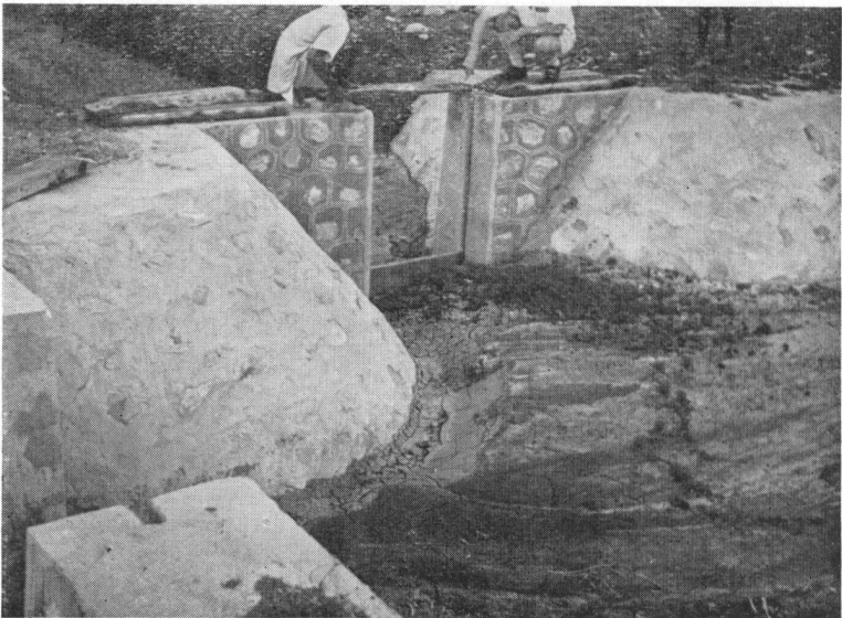
Figure 4. Typical arrangement of two stop log gates, one for inlet water and the other for surplus water
